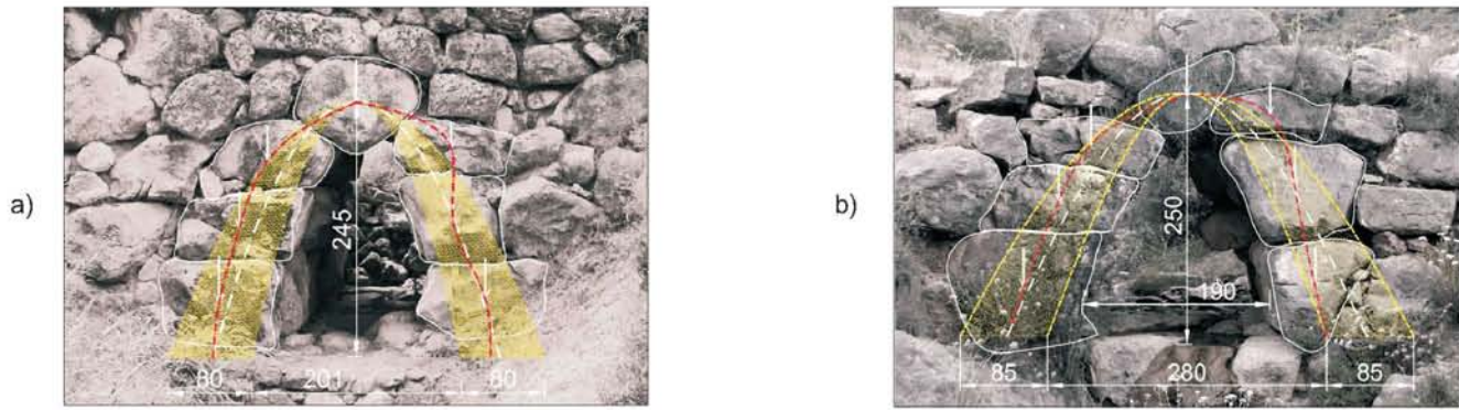
Fig. 11. Hypothetical parabolic arch and its envelope in the arbitrarily defined system visible from the downstream side: a) bridge A, b) bridge B; dimensions in cm
