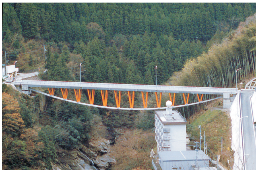
Rys.17. Most ukończony [8] Fig.17. Completed bridge [8]
