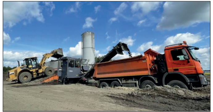
Fig. 4. Wirtgen KMA 220 mobile mixing plant in operation; photo: M. Krasowski
