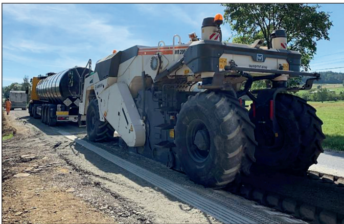
Fig. 3. Wirtgen WR 200i recycler in operation; photo: J. Krasowski
