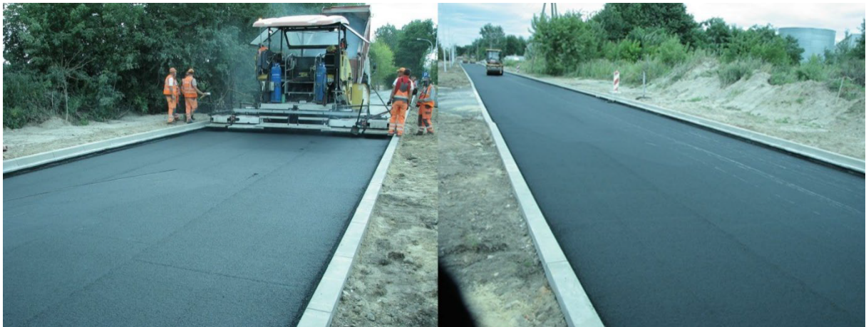
Fig. 11 Pavement construction layer with asphalt rubber binder, Parzniewska Street in Pruszków
