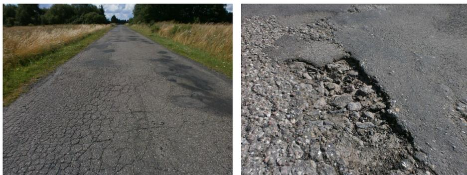
Fig. 1. A bituminous pavement affected by cracking and ravelling
