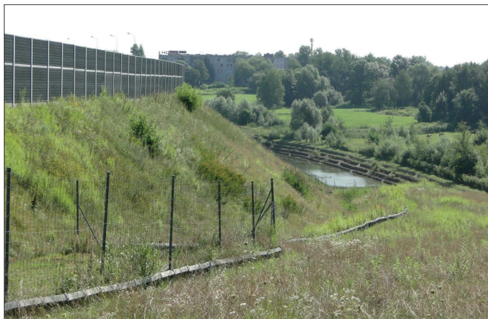
Fig. 8. Storm water retention pond collecting runoff from the highway, situated at the bottom of the deepest closed basin lake on the south side of the A1 Highway, west of the "Bytom" junction
