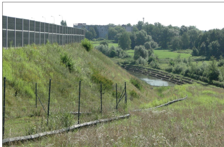
Fig. 8. Storm water retention pond collecting runoff from the highway, situated at the bottom of the deepest closed basin lake on the south side of the A1 Highway, west of the “Bytom” junction
