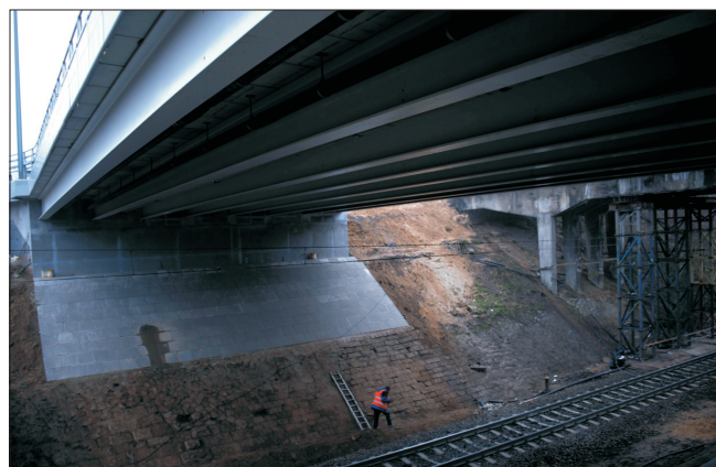
Fig. 2. Superstructure of the viaduct made of HEB800 I-beams (source: J. Czerwiński)
