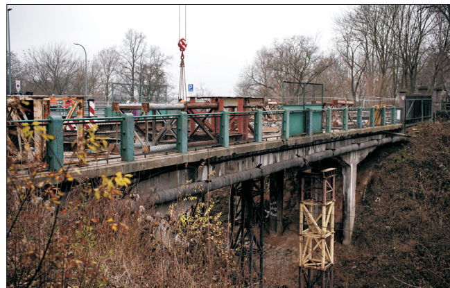
Fig. 3. Demolition of the existing engineering structure (source: J. Czerwiński).
