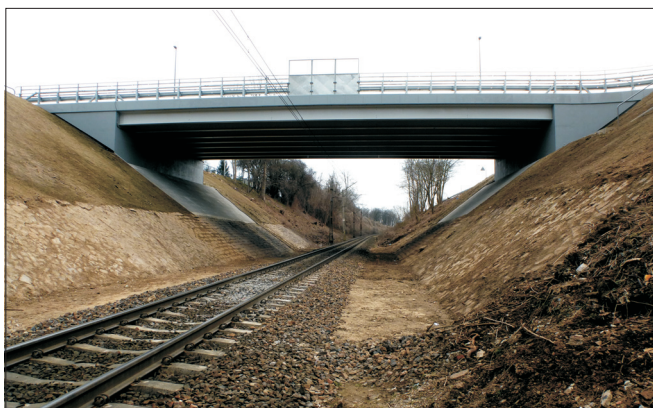
Fig. 1. New road engineering structure over the railway line in Płock
