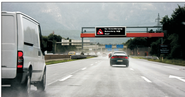
Fig. 4. Example of an integrated variable message sign (IVMS): graphic sign and text board [7]
