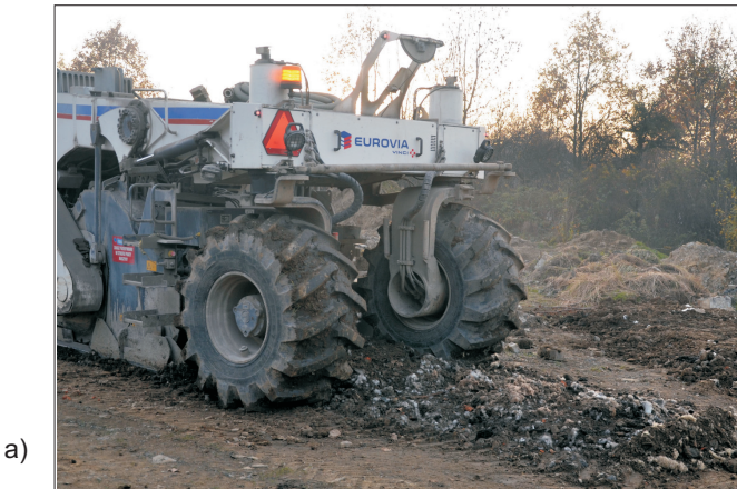
Fig. 1. Installation of the geotextiles: a) mixing of soil with fibres using a road recycler, b) covering of the geotextiles with the fibre-reinforced soil
