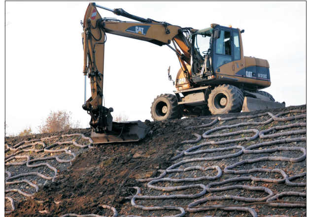
Fig. 1. Installation of the geotextiles: a) mixing of soil with fibres using a road recycler, b) covering of the geotextiles with the fibre-reinforced soil
