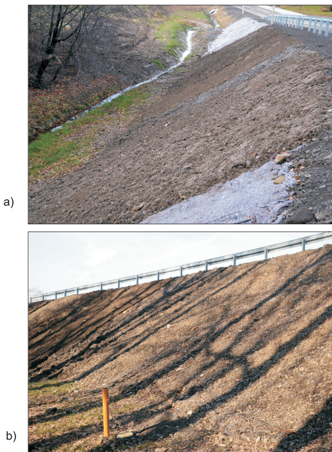
Fig. 2. The protected slope: a) before winter (November 2018), b) after winter (March 2019)
