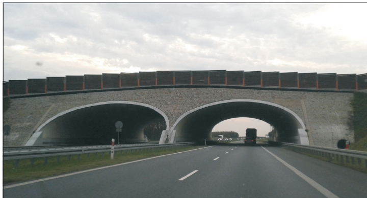
Fig. 1. Wildlife overpass with soil-shell structure on S8 expressway (photo by W. Jasiński, 2017)
