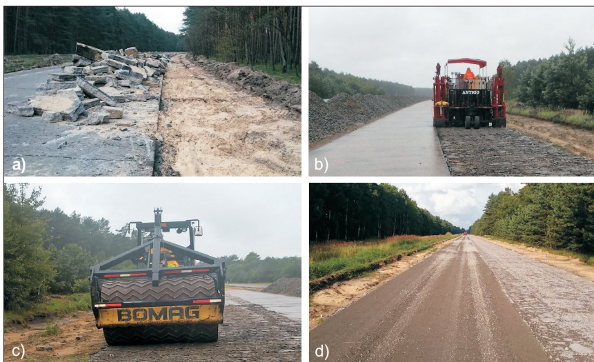
Fig. 7. Stages of building the base-course from the old concrete pavement on DW 142 road: a) removing the emergency lane, b) rubblizing, c) compaction with a 9 t grid roller, d) ready base course
