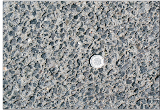
Fig. 2. Exposed aggregate concrete produced using basalt aggregate on the Section A
