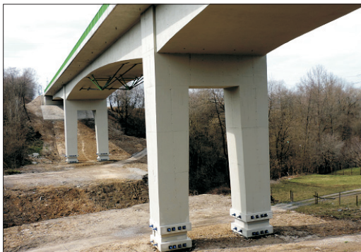
Fig. 14. The bridge substructure and bridge accessory equipment after reconstruction
