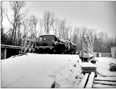
Fig. 5. Variant V of a construction, the DMS-65 bridge with an elongated transverse beam
