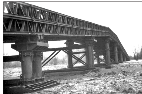
Fig. 4. Variant III of a construction, the SWD-83 flyover
