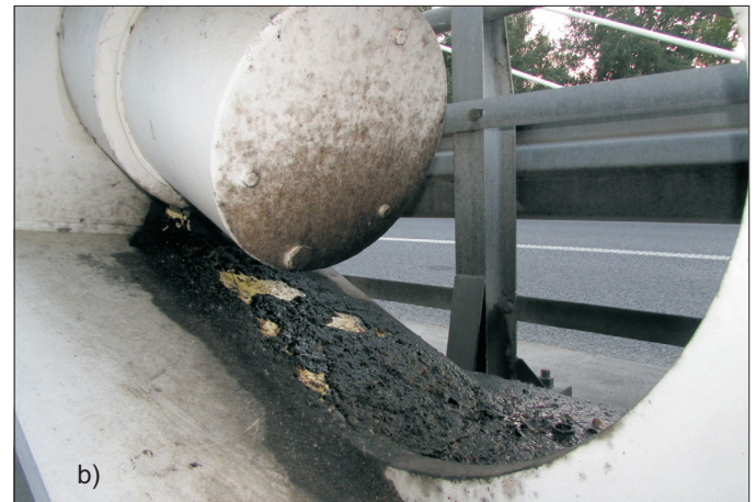
Fig. 5. Dirt: a) graffiti on railings, b) leakage of a substance that protects a cable against corrosion (own photos)
