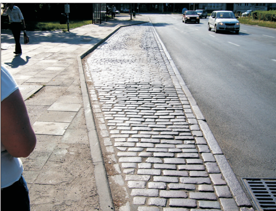
Fig. 7. Pavement laid on loamy soil subgrade
