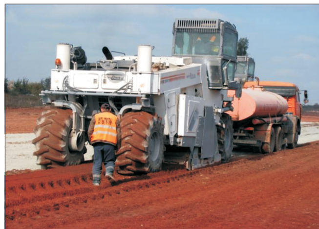
Fig. 2. Stabilization the embankment body composed of coal waste with cement adding
