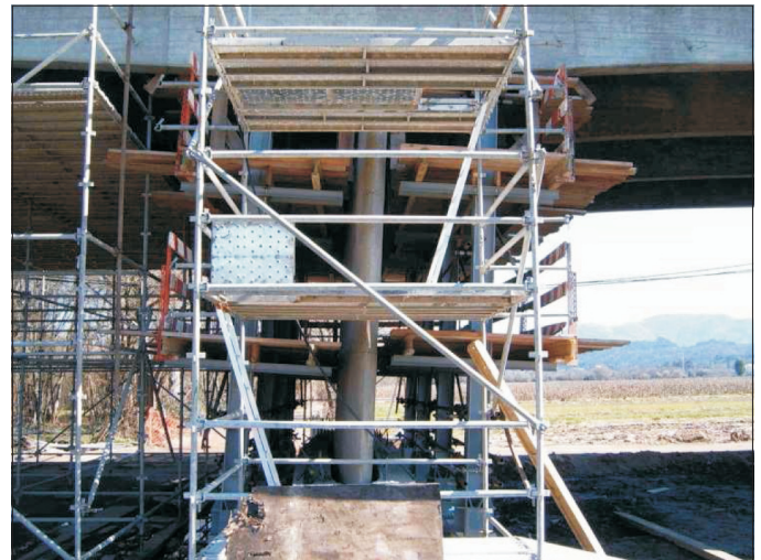
Fig. 4. Example of scaffolding system used to access the test site
