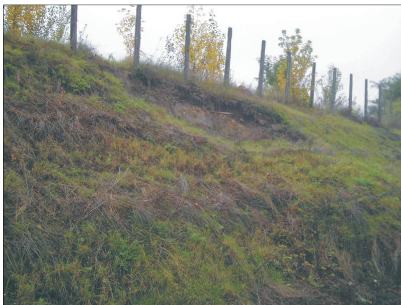
Rys. 6. Obryw mas gruntu na skarpie Fig. 6. Ripping of soil mass on the slope
